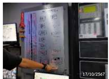
Graphic Annunciator Fire Alarm System
